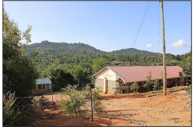
One of the classroom blocks at the school
