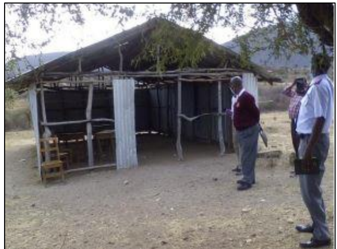
The new classrooms will replace this 'temporary' classroom made from corrugated iron sheets and tree branches.
