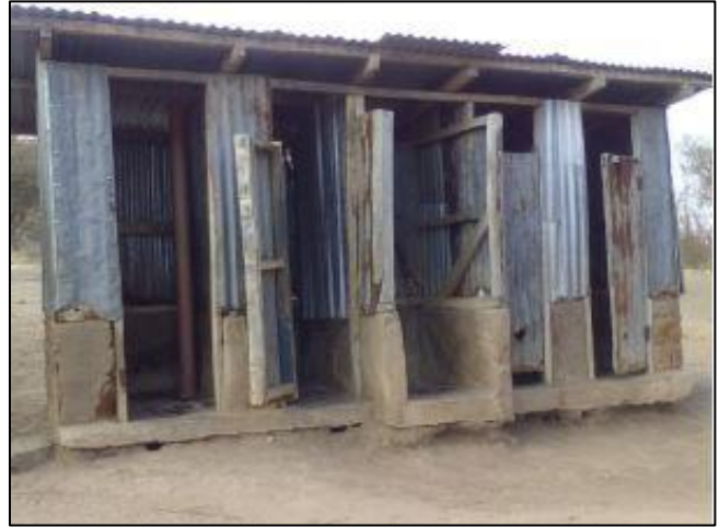
Existing boys pit latrine block.
