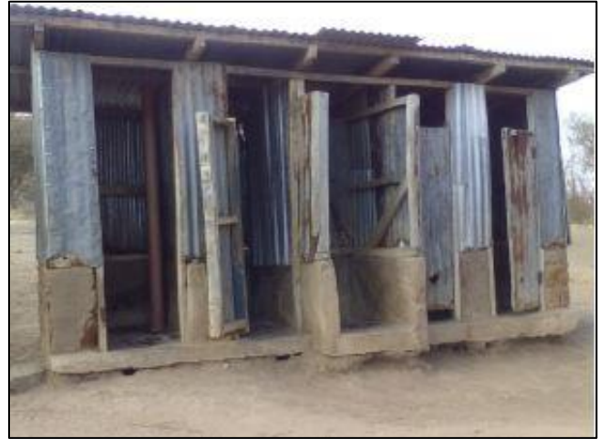
Existing boys pit latrine block.
