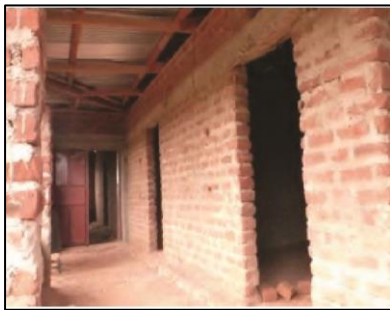
The partially completed clinic:
