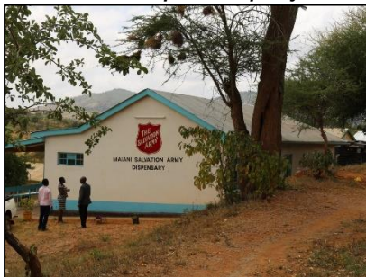
The completed project
