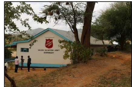
Completed clinic and motorbike for the medic. Inside the clinic medical equipment was provided by The Salvation Army in USA and Australia.
