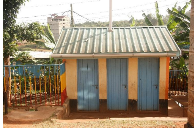
3-cubicle pit latrine at Kibera built with funds from The Kenya Trust in 2019.
