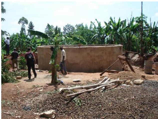
Water tank nearing completion
