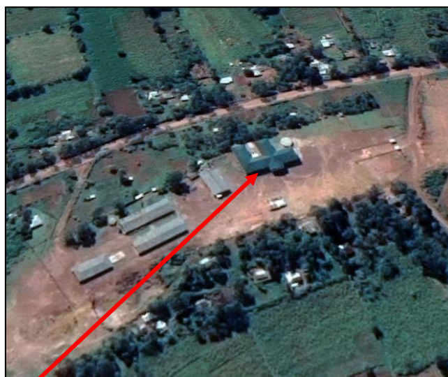
Main Administration Block was recently built with funding from the Kakamega County Government.
