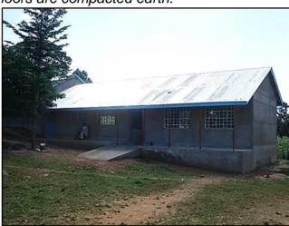
The new construction is of brick and concrete with solid concrete floors. Ramp access is provided for easy access to the classrooms. A total of 4 classrooms are in this block.
