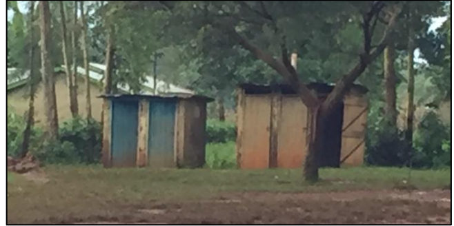
Similar existing latrines at Emurembe:-
