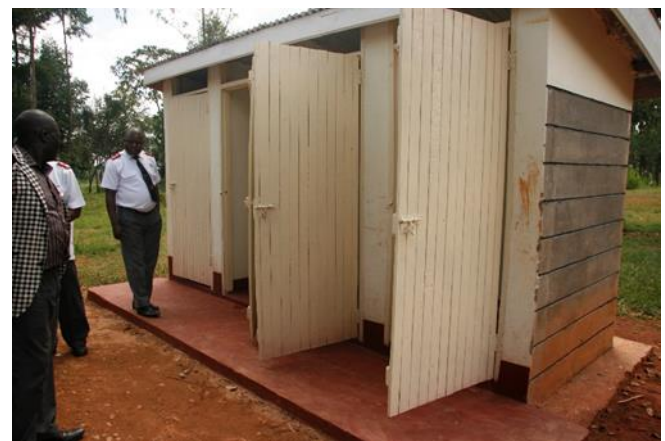
New Construction of latrine block:-
