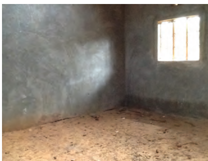
Maiani Medical Centre project
