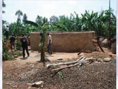
A water project under construction.
