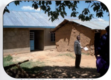
OLD AND NEW BUILDINGS
